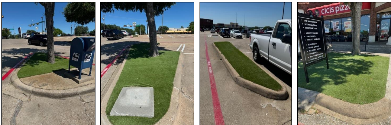
FIGURE 1: PHOTOS PROVIDED BY THE APPLICANT OF THE AREAS WITH ARTIFICIAL TURF
