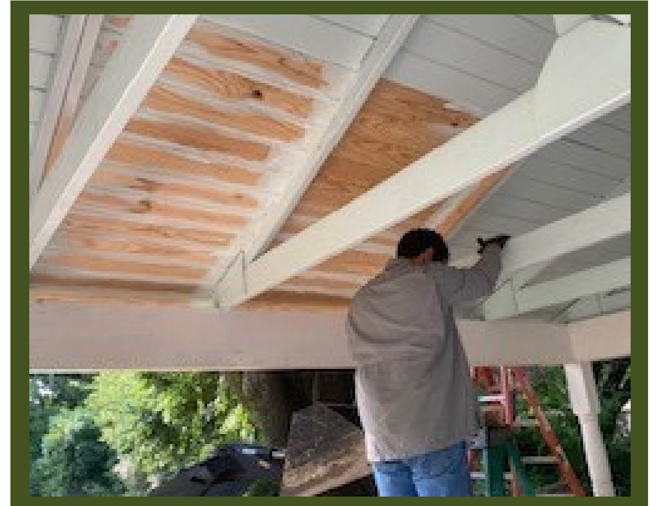
LOFLAND PAVILION REPAIRS
